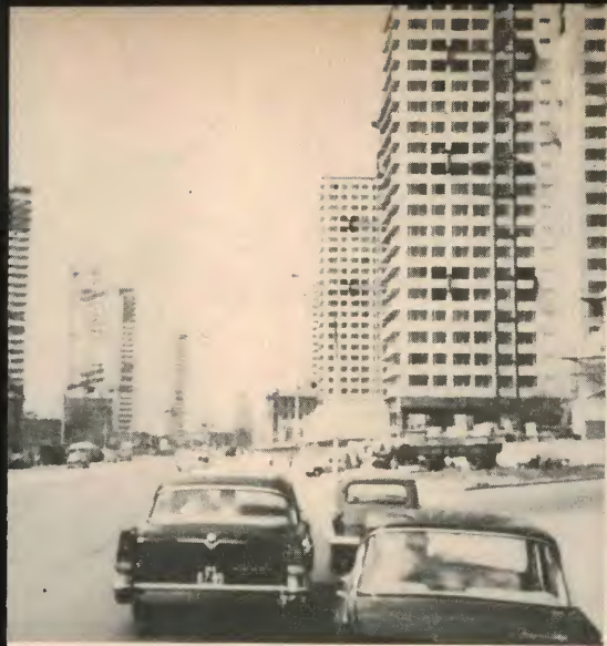
Skyscrapers rise on Moscow's show street, Kalinin Boulevard.
