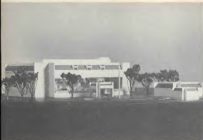
U.S. embassy, Pretoria. This project, which meets the new guidelines for setbacks, also employs a compact overall form with rooftop and high-wall daylighting techniques to minimize exposed glass. (Eduardo Catalano, architect.)
