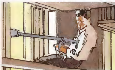
Back out of window with harness secured.
