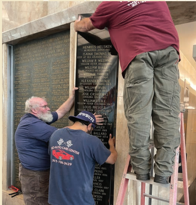
TOP: Master stone mason John Kinnaird (left) and his team install a replacement side panel beside the original 1933 AFSA memorial plaque on the west end of the C Street lobby of Main State. Reinscribing the side panels allowed the 69 new historical names to be incorporated with the existing names in chronological order.
