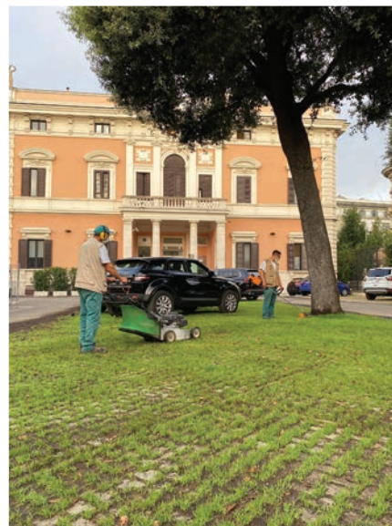
This “green” parking lot made of grass and pavers helps to disperse heat and facilitates rainwater management during storm events.
