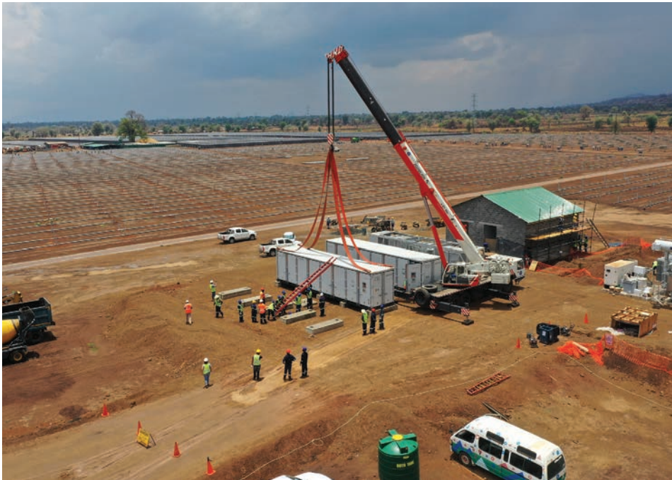
Work is ongoing on the Solar-Plus-Storage power project in Malawi. The 20-megawatt project is the first of its scale there to employ a large-scale battery storage system that allows the plant to provide reliable, renewable energy to the national power grid.
