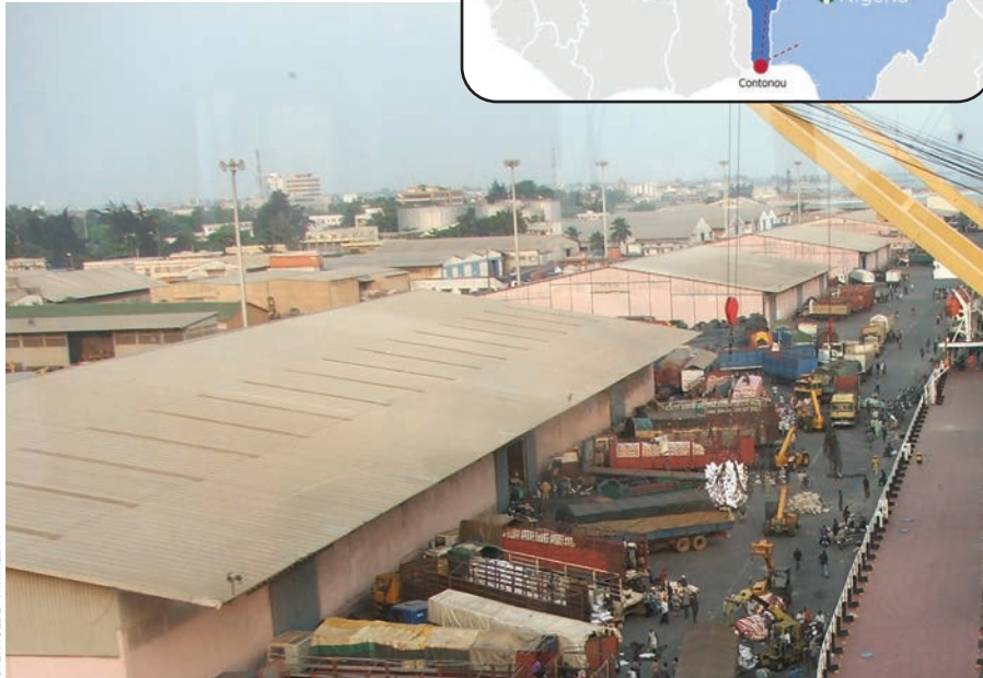
Improvements in operations and infrastructure at Benin's Port of Cotonou supported by the Millennium Challenge Corporation are opening up the economic potential of the region. Inset: Map showing the beneficially affected countries.
