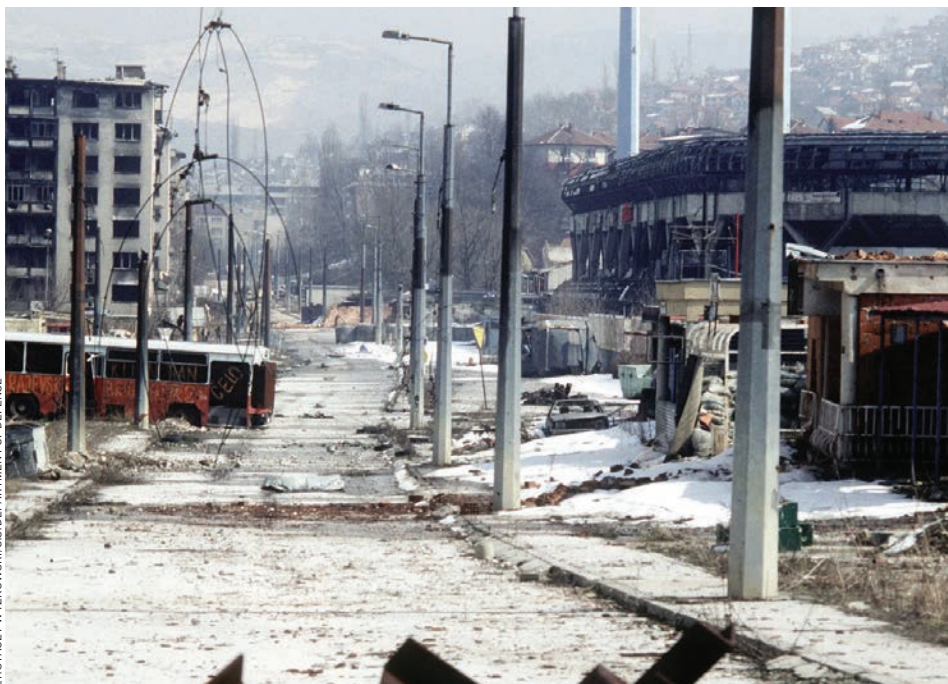
Buildings and vehicles destroyed in Grbavica, a suburb of Sarajevo, Bosnia and Herzegovina, during the Bosnian conflict.
