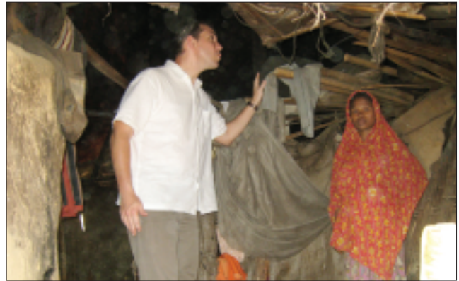
Touring a dilapidated shelter in a Burmese Rongya refugee camp outside of Cox's Bazaar, March 2008.
