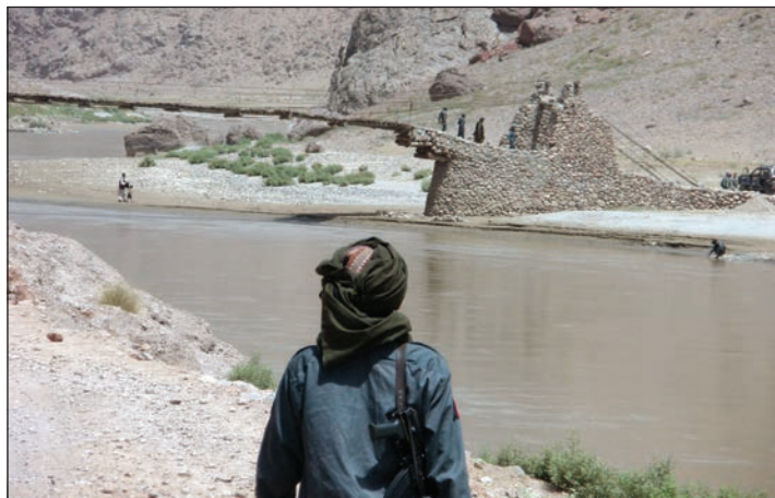
The Taliban funded the construction of this bridge in 1997. Though crude, the structure can be rebuilt every decade and the know-how passed on from father to son.
